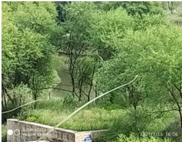
P 31: R. Morwa b/c to Chauri Drain
