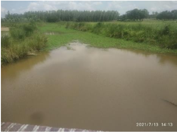
P 3: R. Varuna at Tarhati, Jaunpur bridge
