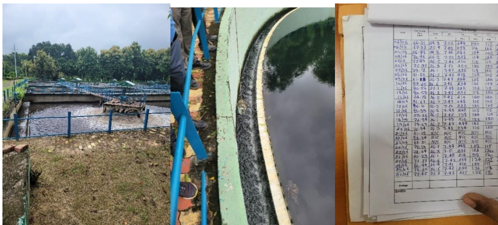
Figure 4.14: 80 MLD Old Dinapur STP
