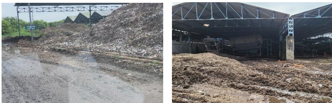
Figure 4.16: Existing Solid Waste Treatment System
