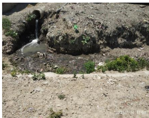
P 24: Unknown Drain d/s Narokhar drain
