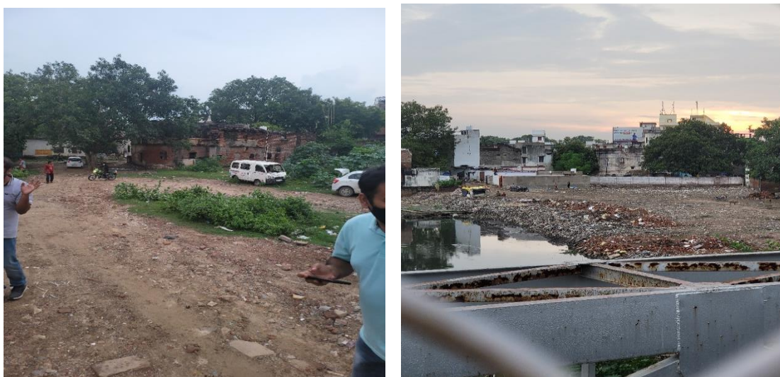
Figure 4.13: Ravinder Puri Culvert as Possible Location for New STP at Assi
