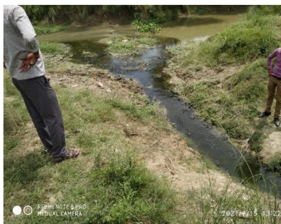
P 36: Barbuspur Drain
