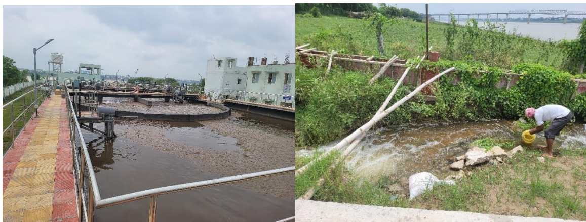
Figure 4.15: 10 MLD Ramnagar STP
