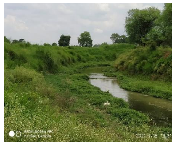
P 30: R. Morwa a/c to Barbaspur Drain
