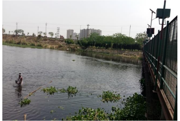
U/s River Hindon –Khareda Drain
