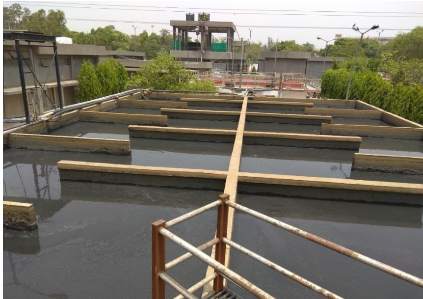
Figure 8: Pre-Chlorination tank at CETP, Mayapuri
