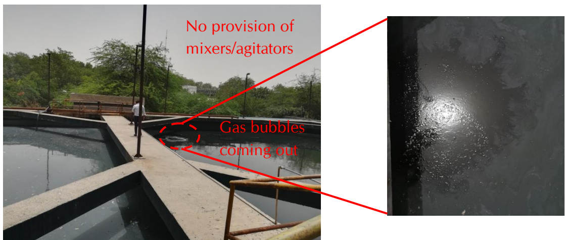
Figure 3: Equalization tank at CETP, Lawrence Road
