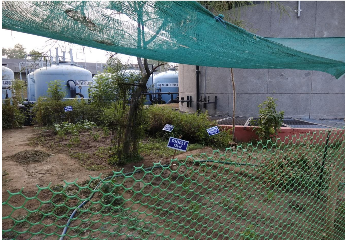
Figure 24: Treated effluent from Mayapuri CETP used for irrigation of vegetables.
