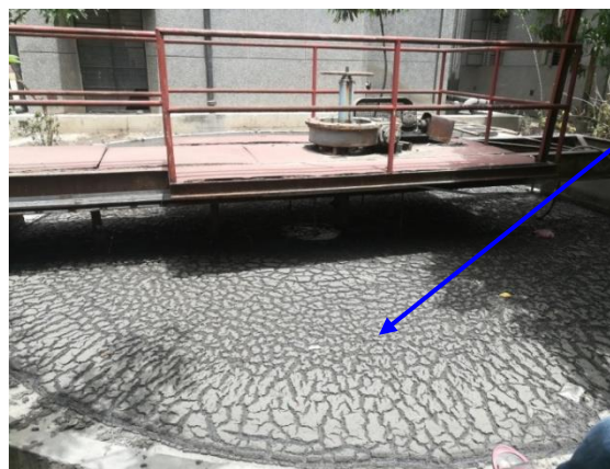
Figure 7: Floating sludge of sludge thickener at CETP, GT Karnal Road
