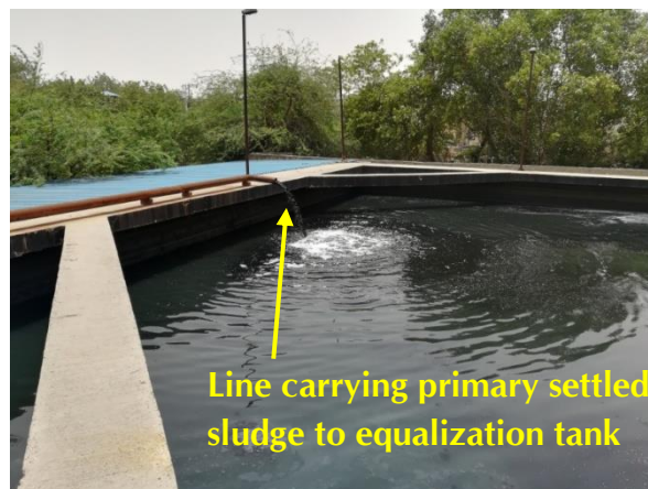
Figure 3: Equalization tank at CETP, Lawrence Road
