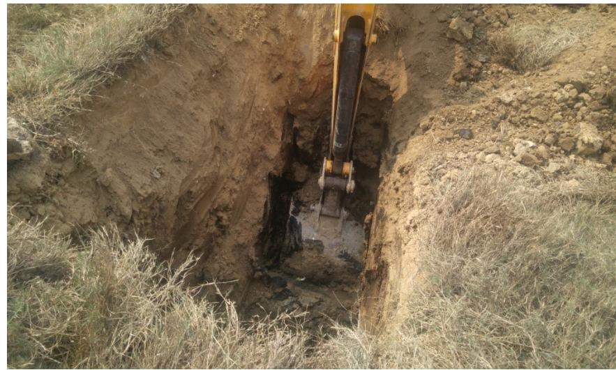
Soil layer at depth of 9 feet having colour of sludge
