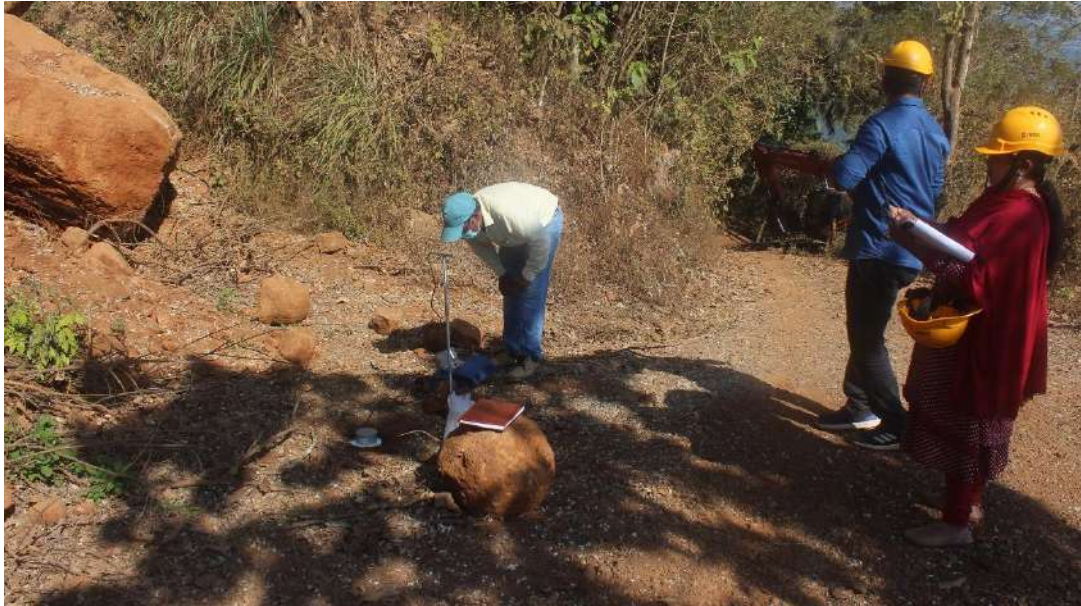
Plate 5.9.5. View of vibration monitoring behind blast face (towards Sri devi Temple)
