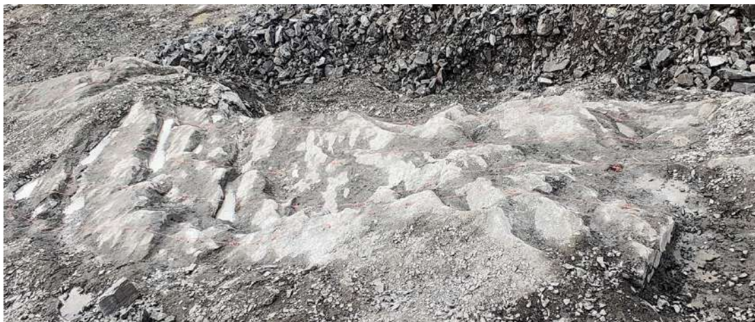
Plate 5.4.10. View of blasting patch, ready to fire
