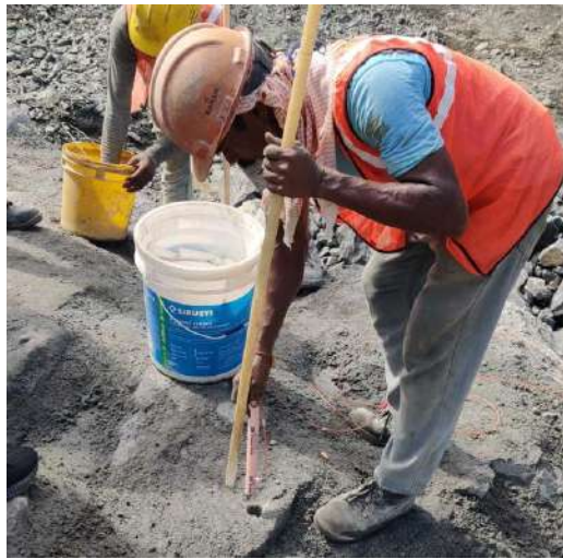
Plate 5.4.9. Charging of explosive into the blast hole and stemming of the charged blast hole
