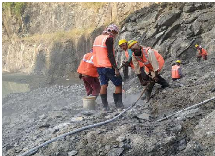
Plate 5.1.4. Drilling of blast holes using Handheld Jackhammer drill machine
