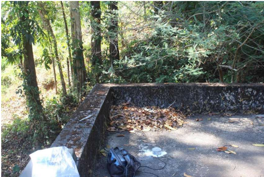
Plate 5.9.8. View of vibration monitoring on the roof of the house Sri Ravi
