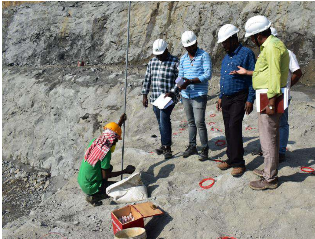
Plate 5.5.9. Stemming material (coarse sand) to fill the blast hole
