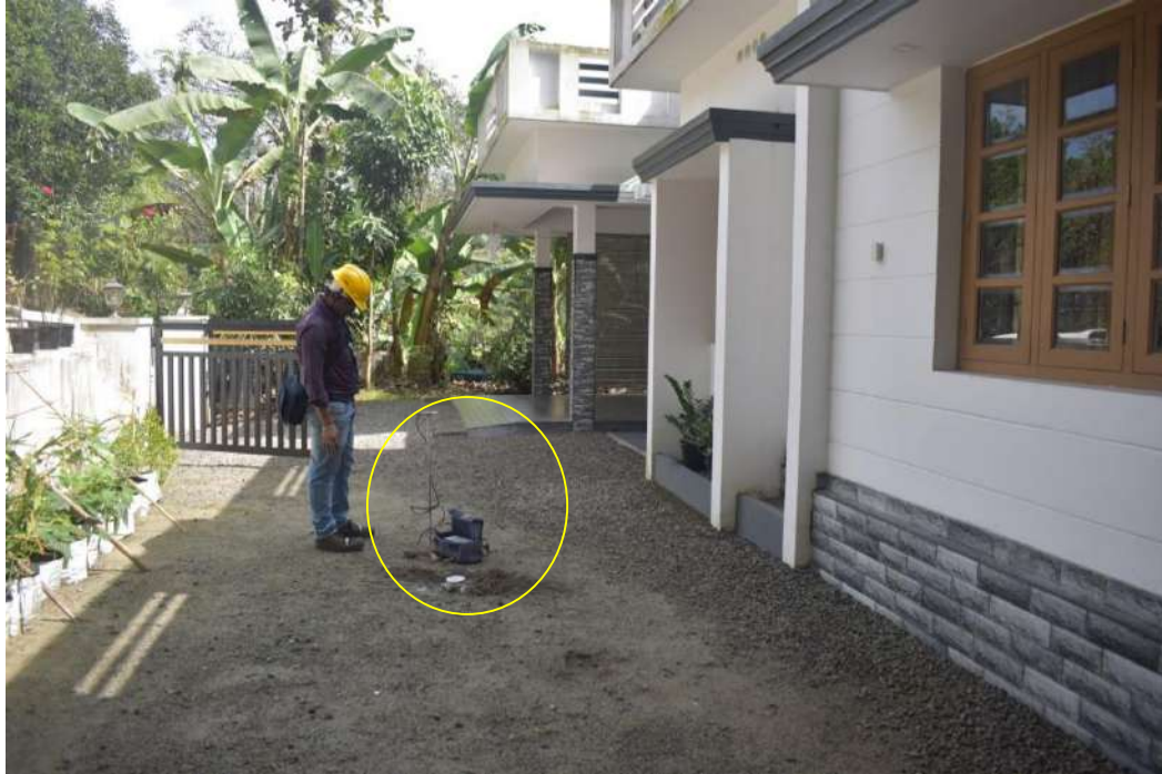
Plate 5.4.15. Monitoring of ground vibration and air overpressure at Jeans' house
