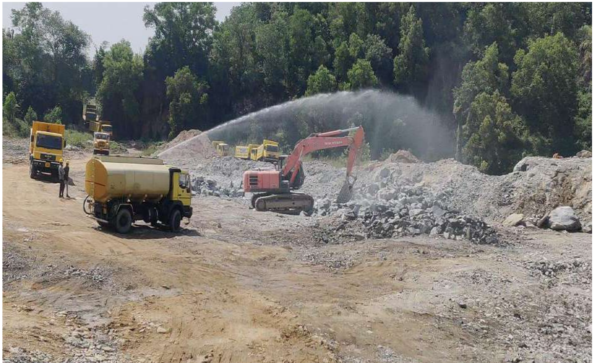
Plate 5.3.10. Water sprinkling arrangement to minimise dust generation during blasting
