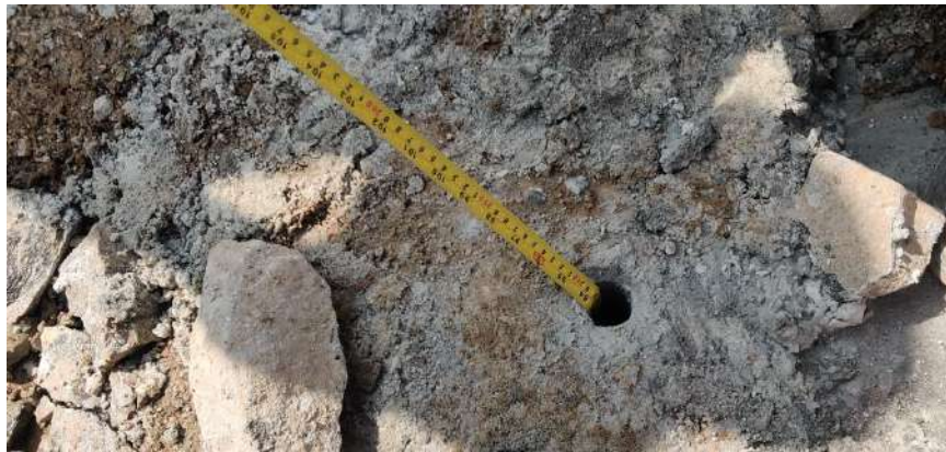
Plate 5.3.5. Measurement of hole depth before charging of holes for correct placement of explosive and to ascertain the required top stemming
