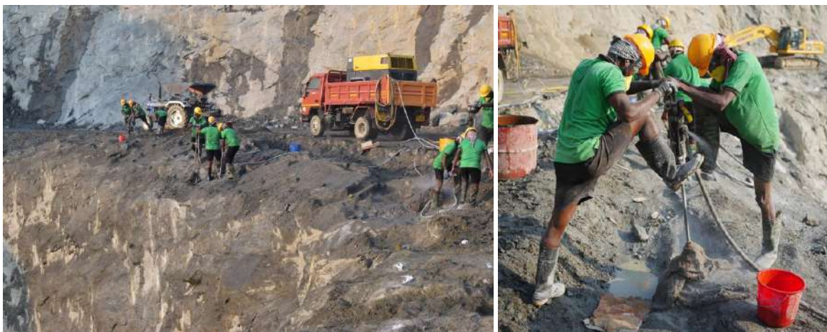
Plate 5.5.7. Drilling of blast holes at Rubble Stone Quarry
