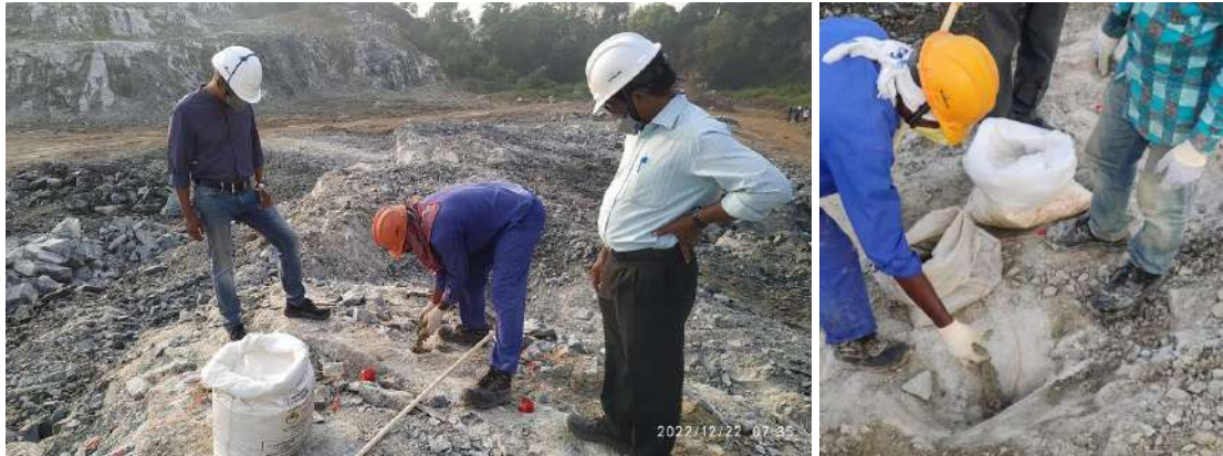
Plate 5.3.7. Stemming of blast hole using coarse sand mixed stone chips
