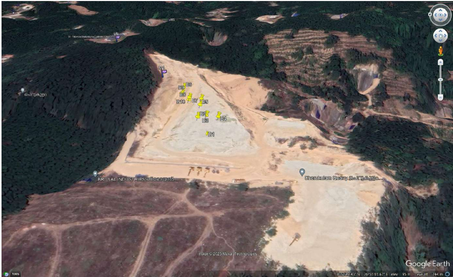
Figure 5.2.1. Google map showing locations of the experimental blasts at granite building stone quarry of Muhammad Roshen, Kollam District
