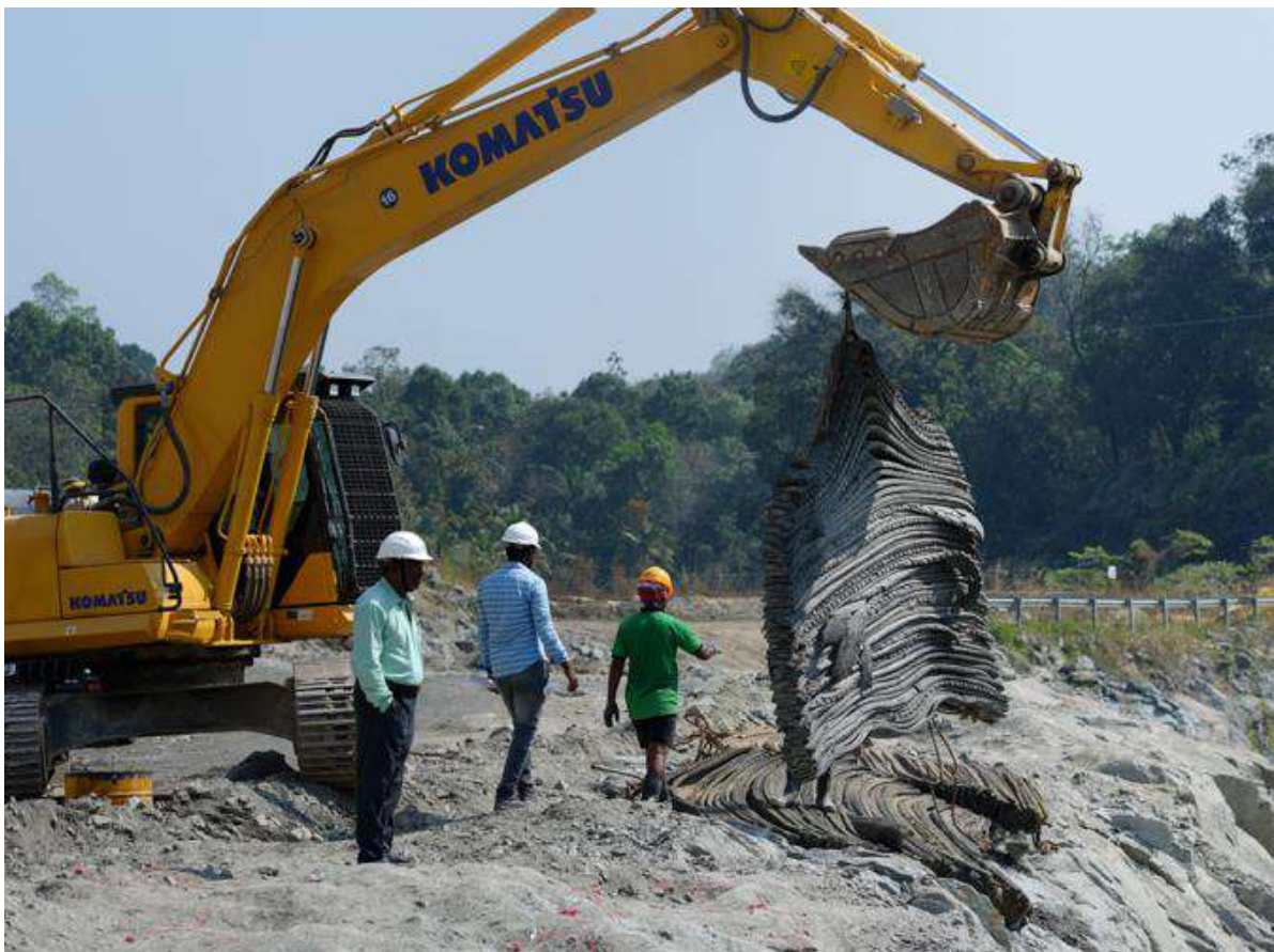
Plate 5.5.10. Muffling of blasting patch using blasting mat
