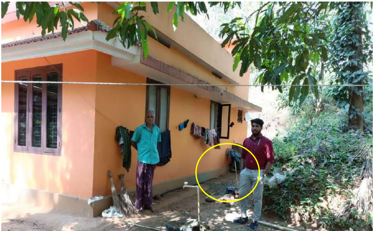
Plate 5.7.6. View of vibration monitoring at the house of Shri Chako P. K. (House no. 124)
