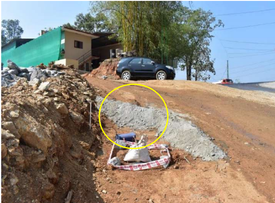
Plate 5.5.13. Monitoring of ground vibration and air overpressure near mine canteen
