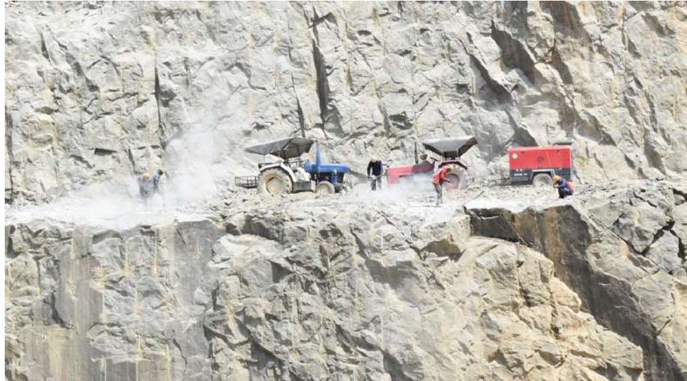
Plate 5.6.6. View of drilling of blastholes
