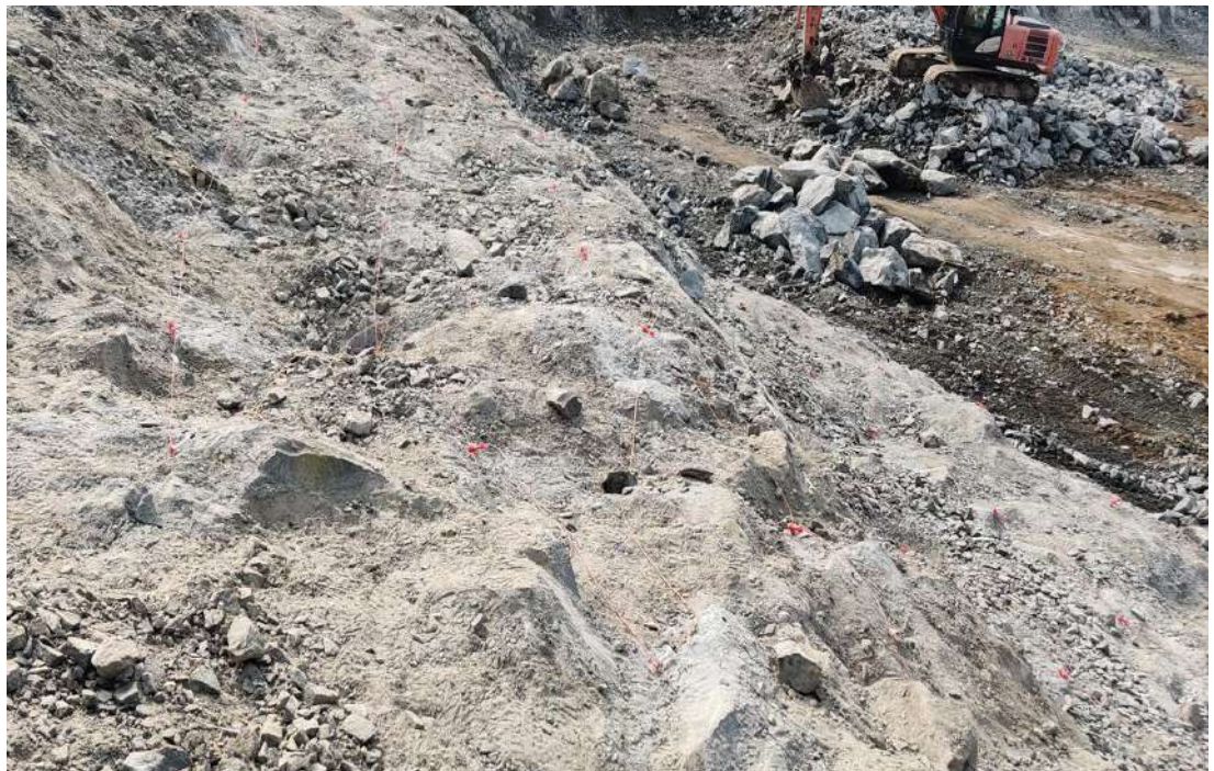
Plate 5.3.8. View of ready to fire blasting patch
