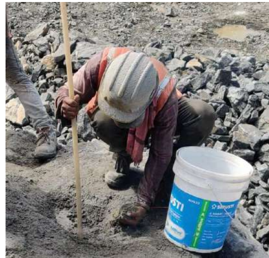
Plate 5.4.9. Charging of explosive into the blast hole and stemming of the charged blast hole
