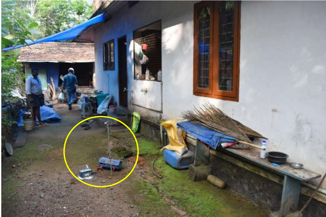
Plate 5.6.13. Monitoring of ground vibration and air overpressure at Shiv Bhavan
