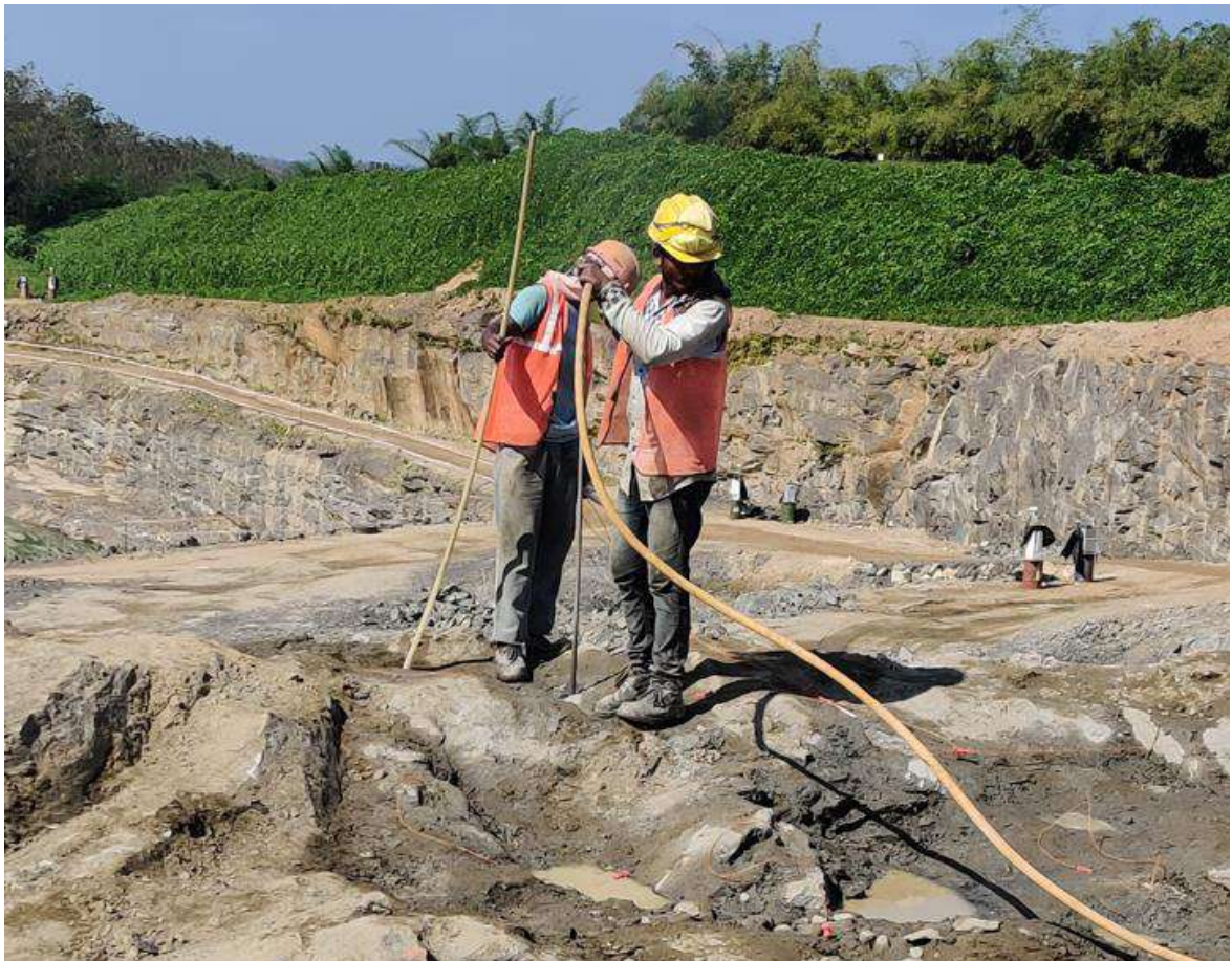
Plate 5.4.6. Arrangement to de-water the blast hole prior to charging of explosive
