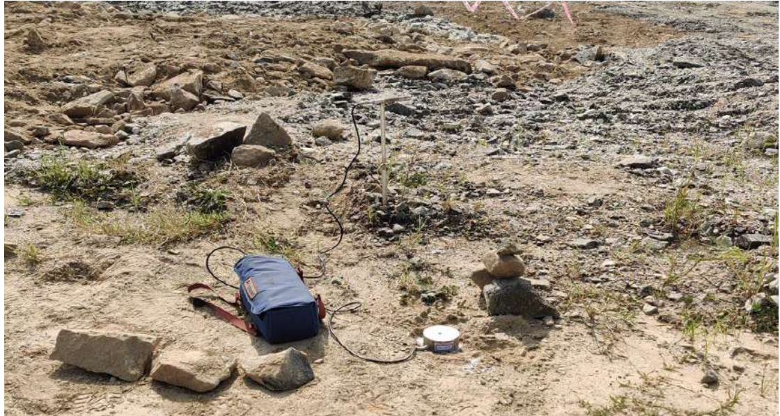
Plate 5.3.17. View of vibration monitoring at backside of free face towards the west direction
