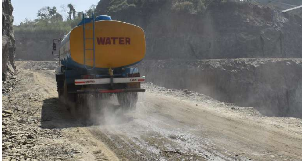
Plate 5.6.8. Water sprinkling arrangement to minimise the dust generation during blasting
