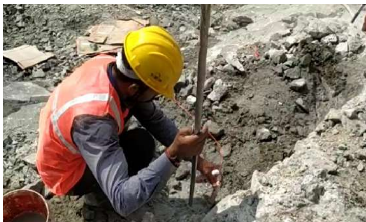
Plate 5.1.5. Charging of holes at Granite Building Stone Quarry
