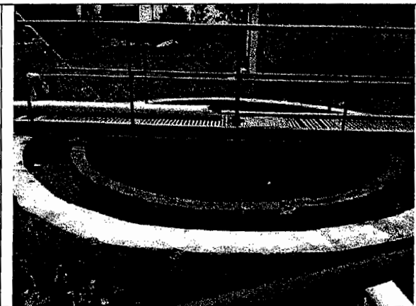
Fig: Clarifier with no effluent
