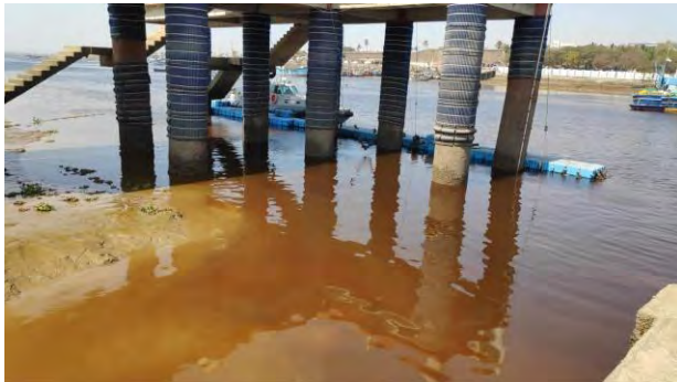
River Damanganga – Daman Jetty
