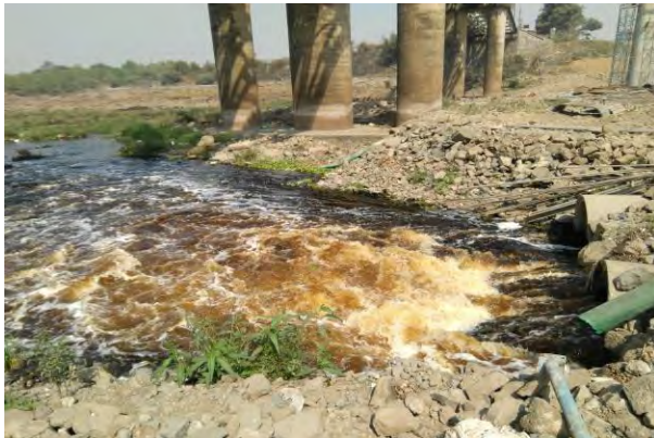
Constriction of River Damanganga flow due to Bridge Construction
