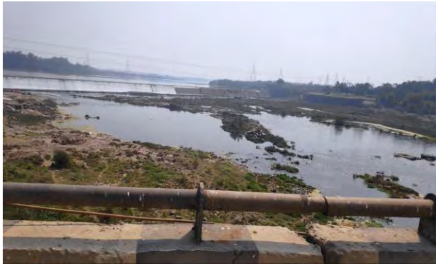
GIDC Weir view from NH-8
