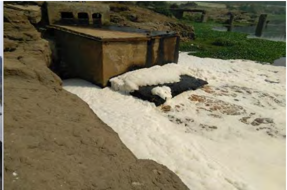
CETP Discharge into River Damanganga
