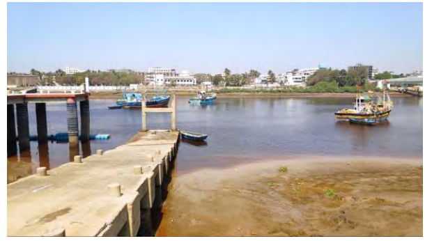
River Damanganga – Daman Jetty
