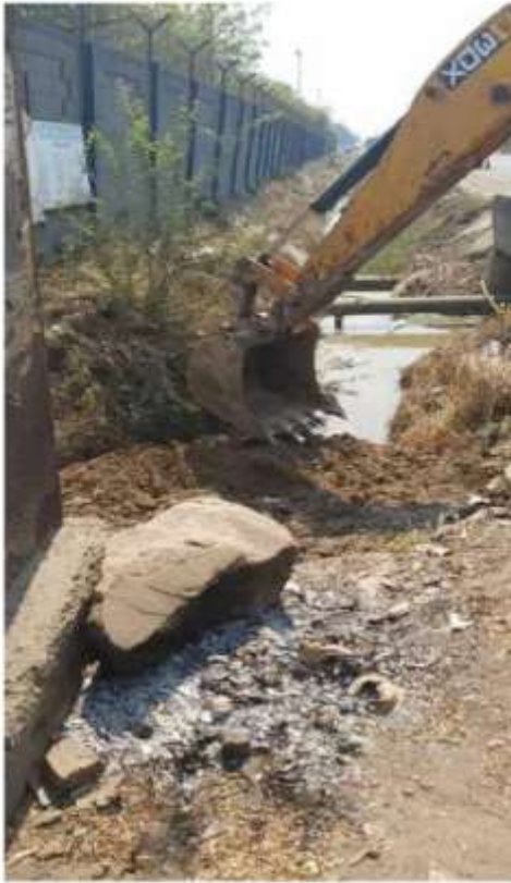
Bund wall making with JCB in nearby storm water drain.
