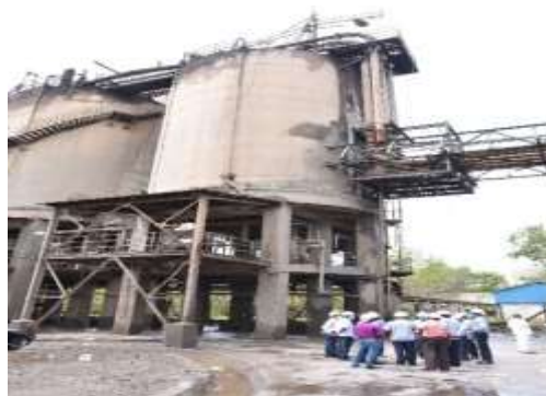
Figure 11 Silo for fly ash collection
