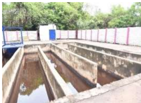
Figure 9 Settling tank
