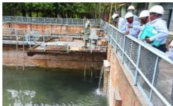
Figure 8 Neutralization Tank
