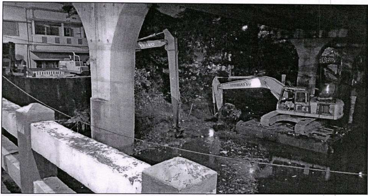
Dredging of Tolly's Nullah (Adi Ganga)
