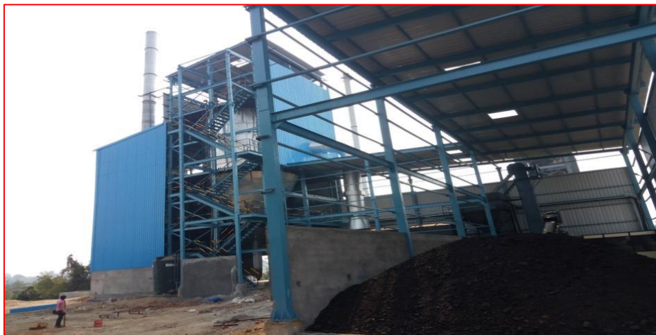
Photo-6 Spray dryer (for concentrate from Common MEE)
