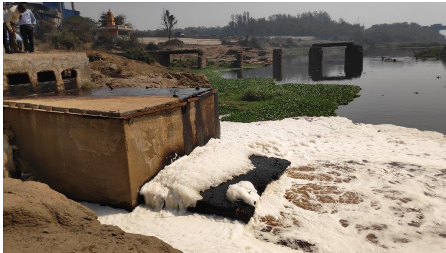
Photo-8 Treated effluent discharge in to the river
