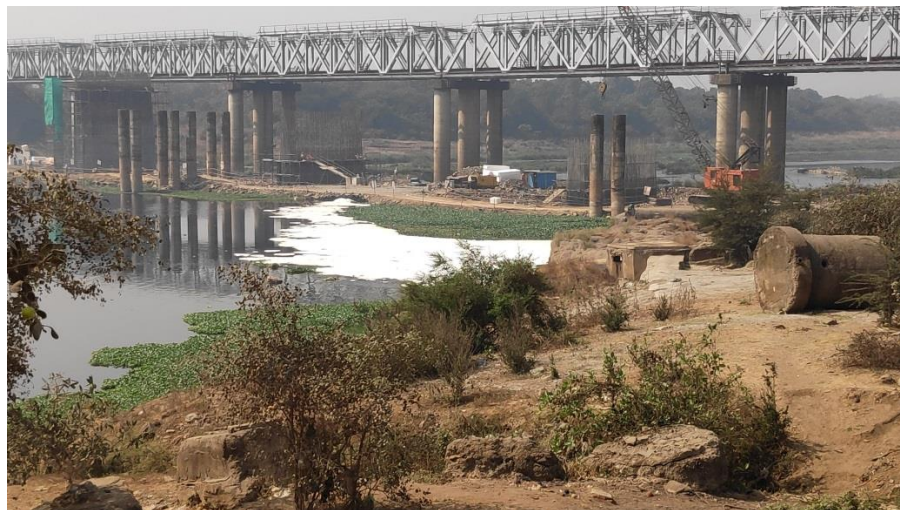
Photo-9 Treated effluent discharge in to the river
