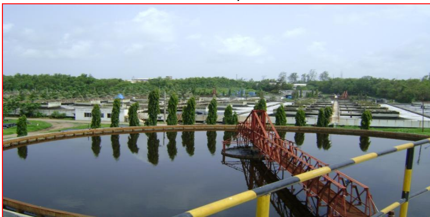
Photo-3 Secondary Clarifier
