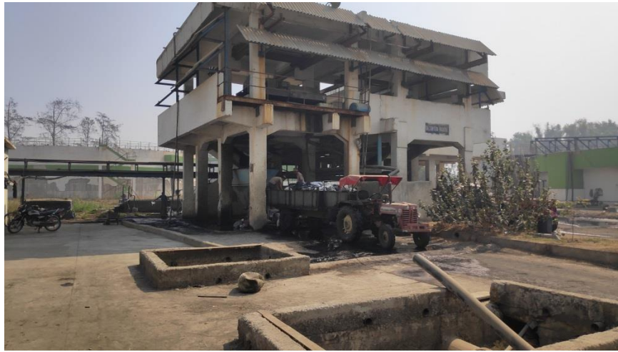
Photo-4 Sludge dewatering (centrifuge)
