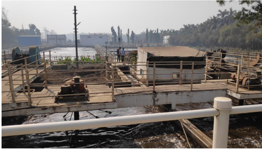
Photo-1 CETP Vapi- Grit Chamber & Equalization Tanks
